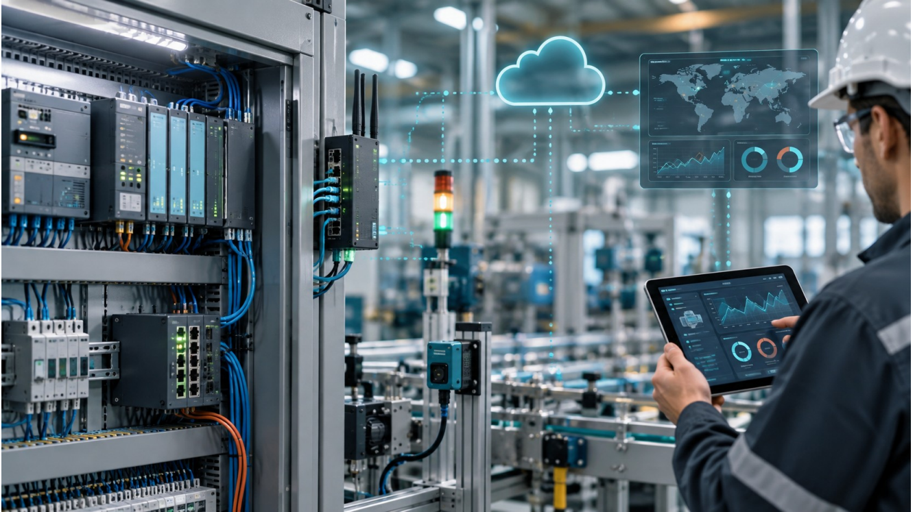
Illustrative connected-factory and edge-monitoring environment.
